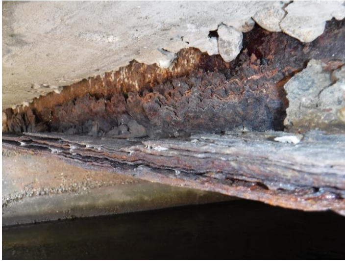
Fascia Beam – Significant Section Loss
