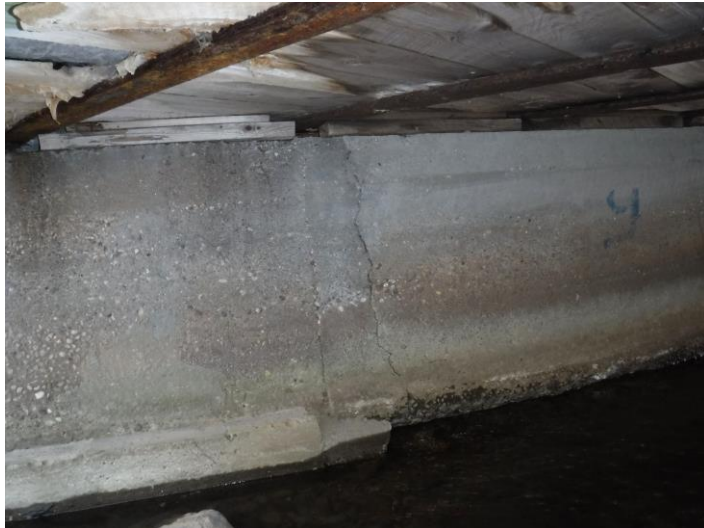
Abutment - Undermining with Vertical Crack
